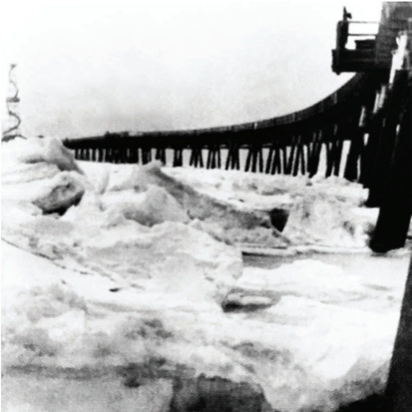
Figure 7. Ice ridges on the approaches to the piers of the Izberg-Sea oil field in February 1953 (Photo from the archive of "Rosneft-Dagnefte" OJSC)
